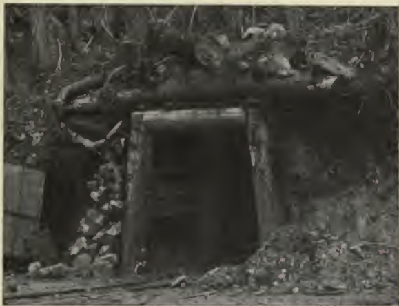
FIG. 98.—MOUTH OF A TUNNEL
